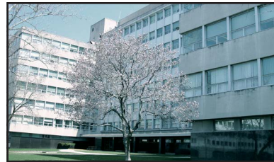
Stratton Building the TRS office from 1955 - 1966
